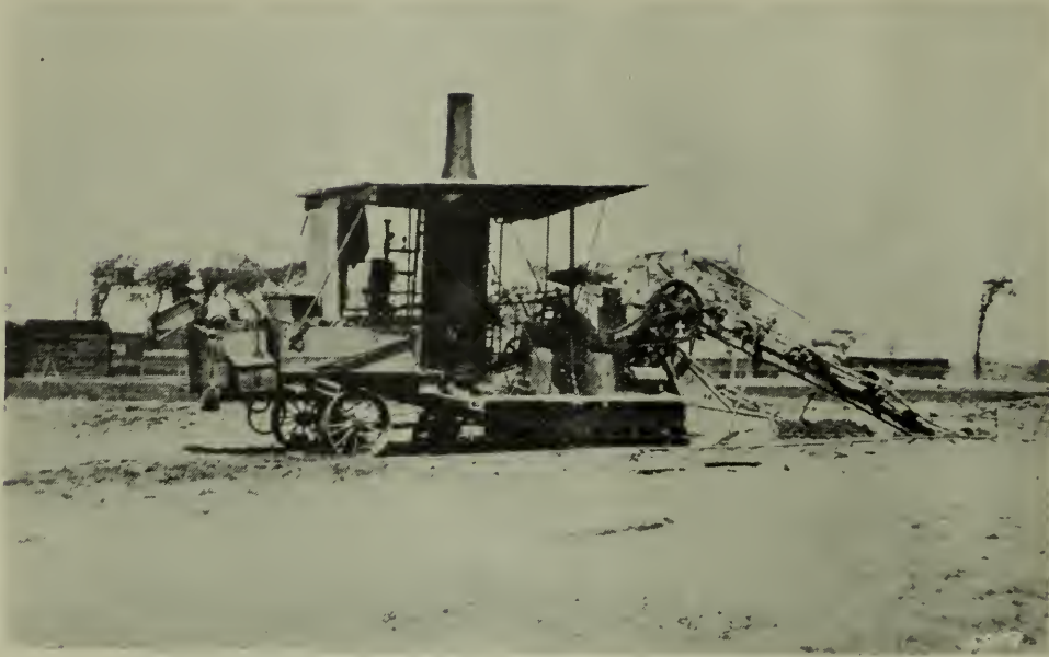
FIG. 5. SIDE VIEW OF A STEAM DIGGER CUTTING A DRAINAGE TRENCH.
